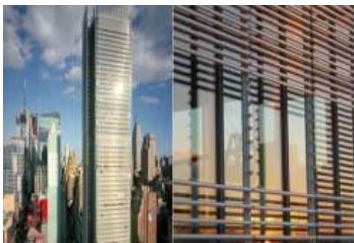
Fig. 10: New York Times Building Fig 11: Detail of ceramic shading elements Source: www.brianrose.com Source: architecture.co
