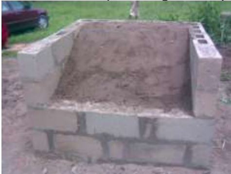
Plate 1: Basement for metal plate
