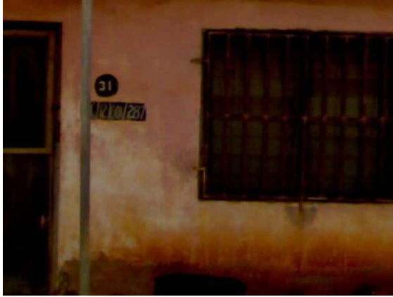
Plate 5: Picture Showing Paint Discolouration in One of the Building in Shagari Estate
