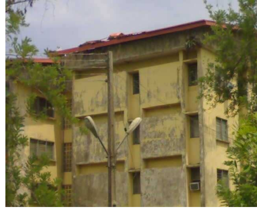
Plate 6: Picture Showing Discolouration in One of the Building in Alagbaka Estate
