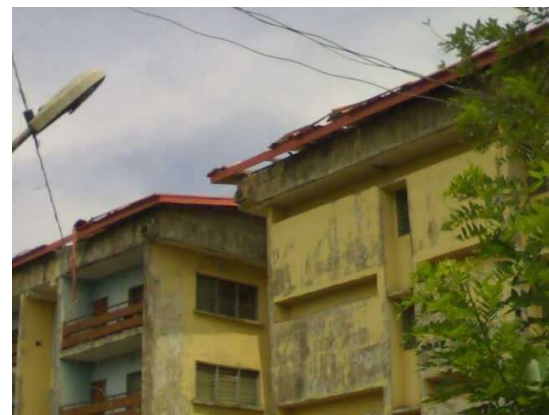
Plate 8: Picture Showing a Bad Portion of Roof in Some of the Buildings in Alagbaka Estate
