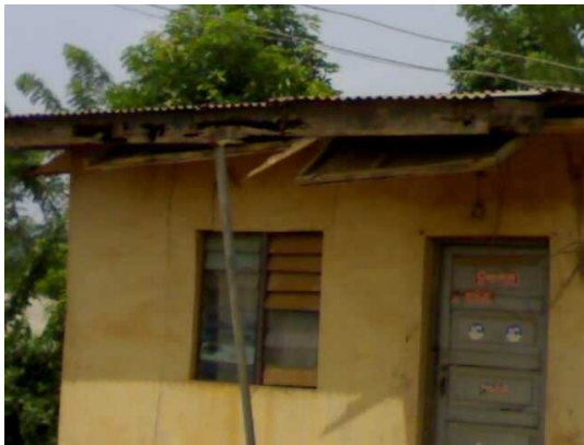
Plate 3: Picture Showing Bad Portion of the Ceiling in One of the Buildings in Shagari Estate
