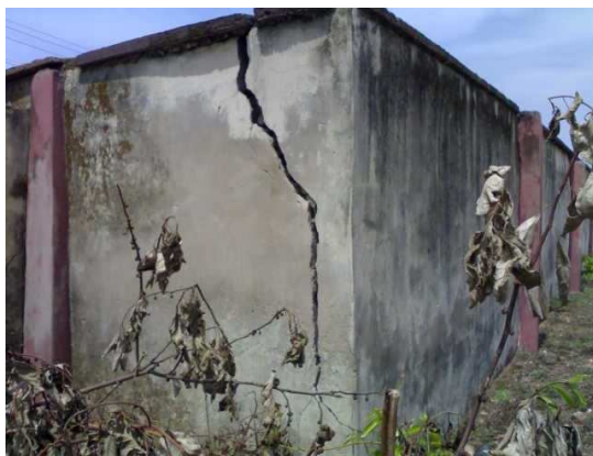
Plate 7: Picture Showing a Deep Crack on the Wall of a Building in Alagbaka Estate
