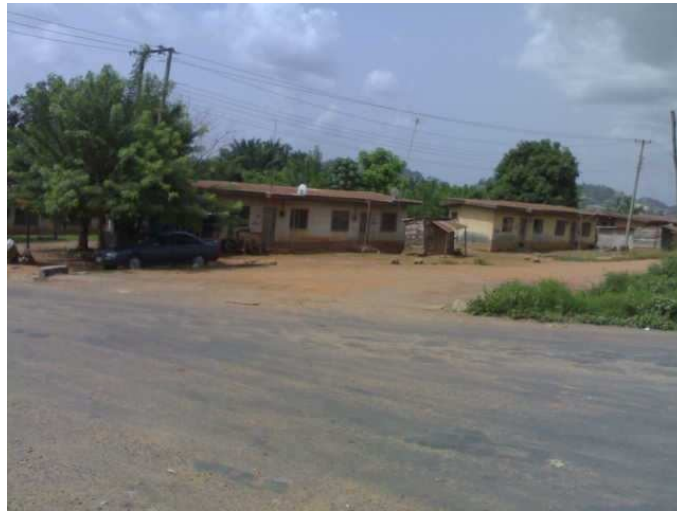
Plate 2: Picture Showing Some of the Buildings in Shagari Housing Estate, Akure.
