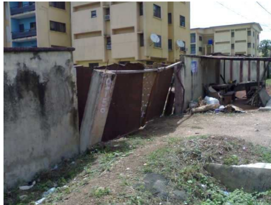
Plate 9: Picture Showing a Bad Portion of the Fence of a Building in Alagbaka Estate
