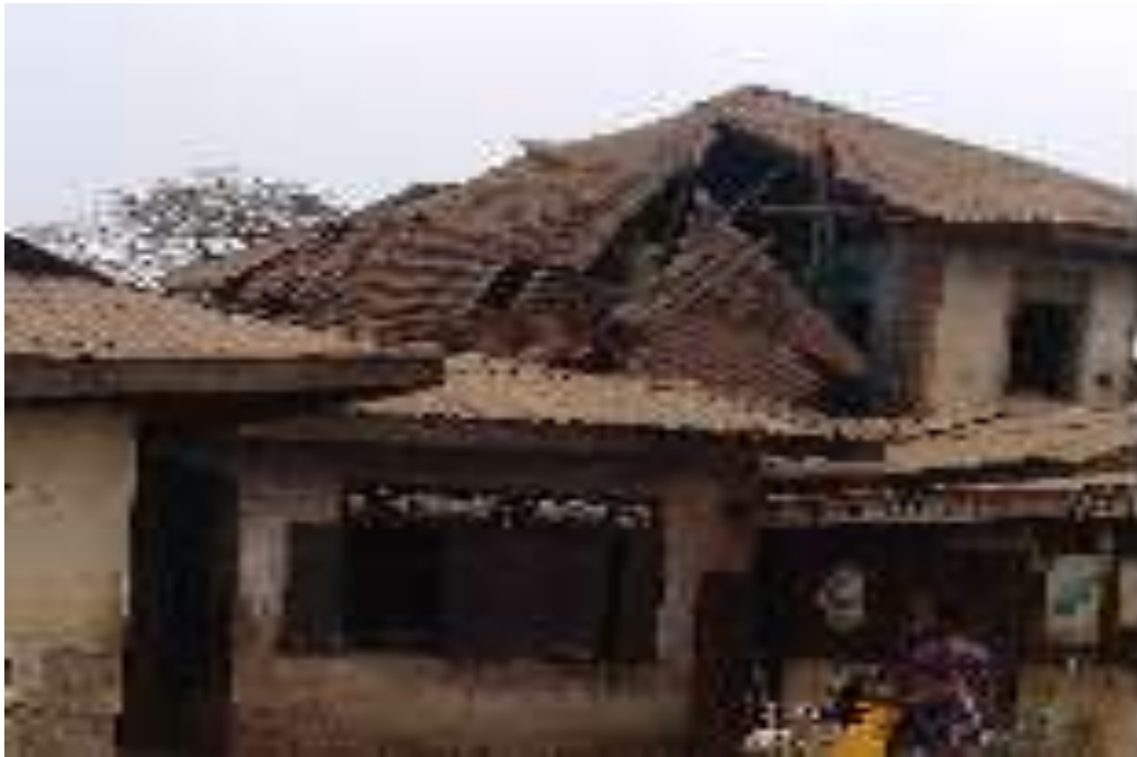
Plate 2. : A Very Poor Condition of Wall and Roof in Beere
