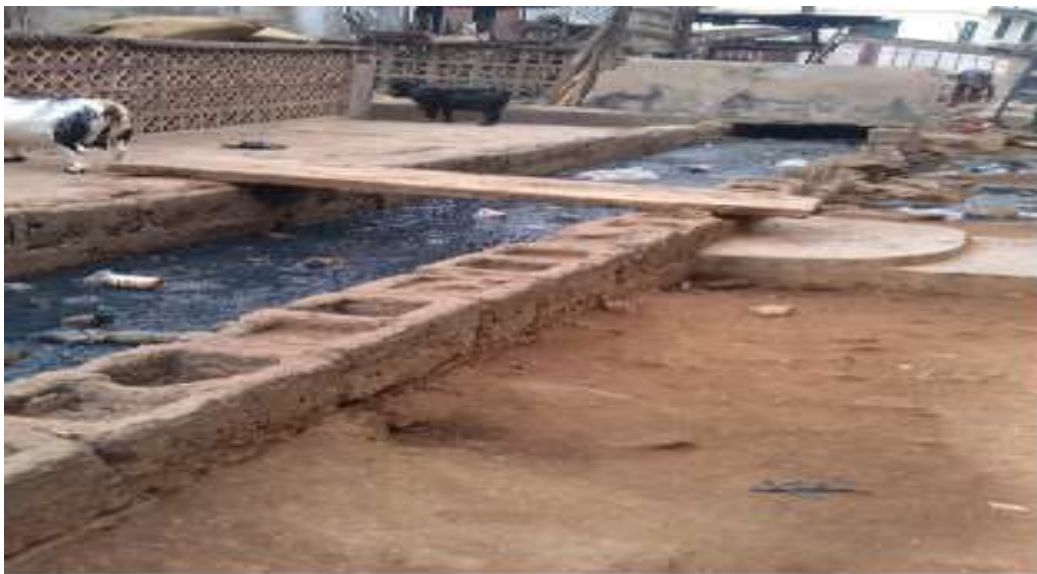
Plate 1: Blocked Drainage System in Samonda.
