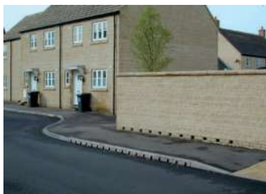
Figure 5: Drainage Relief Openings
