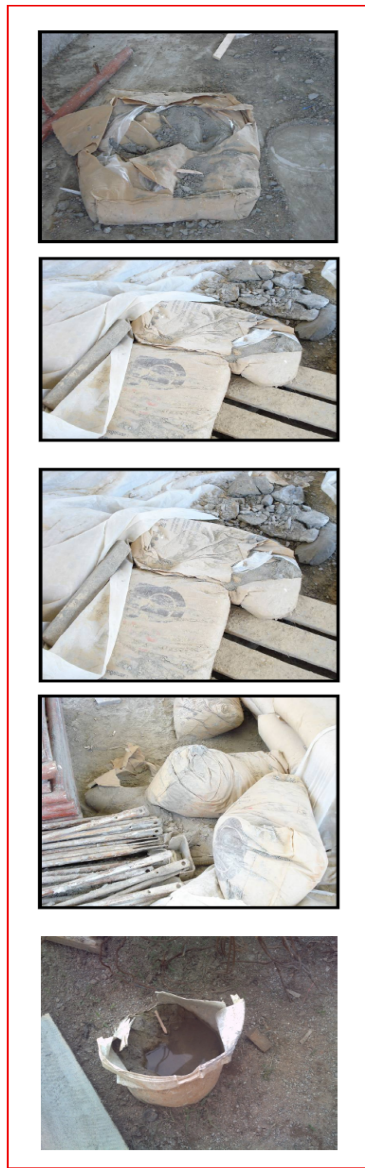
Fig 7a: Ways in which Cement is Wasted on Construction Sites
