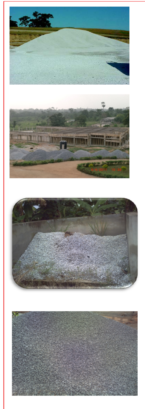
Fig. 6b: Recommended Ways of Storing Materials for Concrete Production on Site
