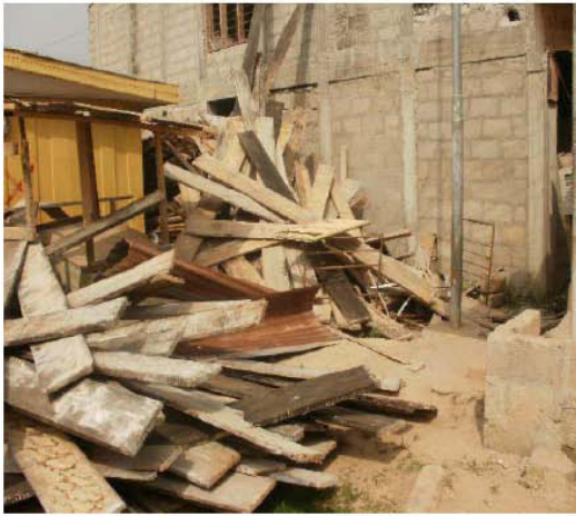
a) Dismantled formwork boards
