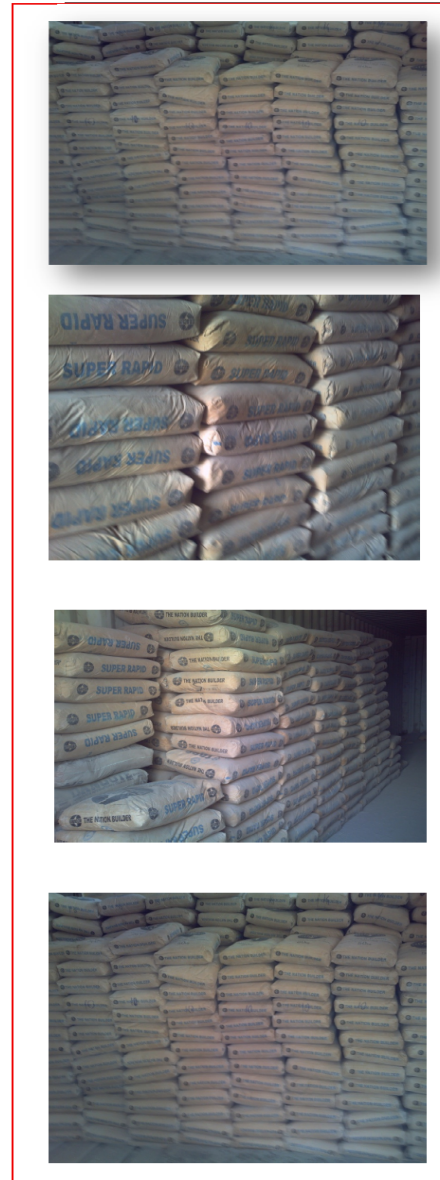
Fig 5b: Recommended Ways of Storing Cement on Site
