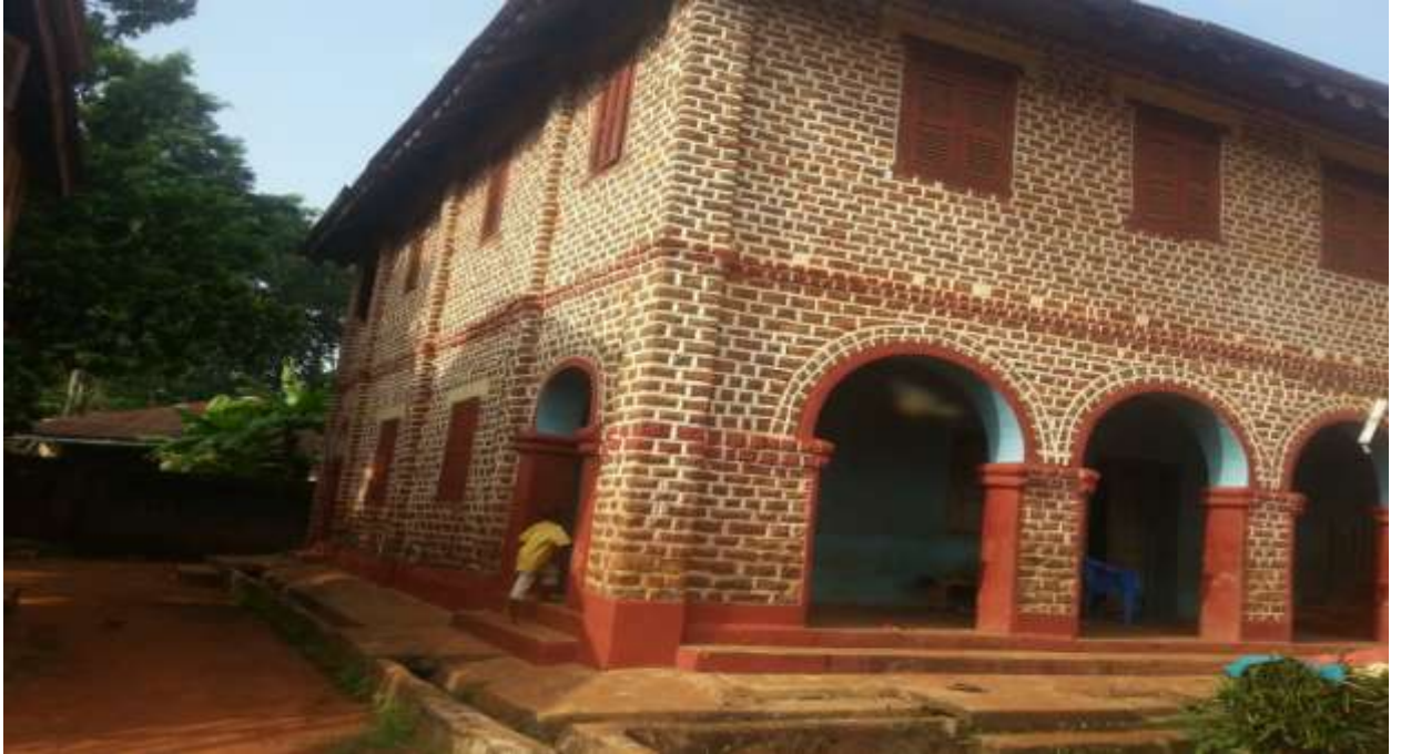
Plate 1: A building in a Traditional Ruler's palace in which walls were constructed with locally available stone.
