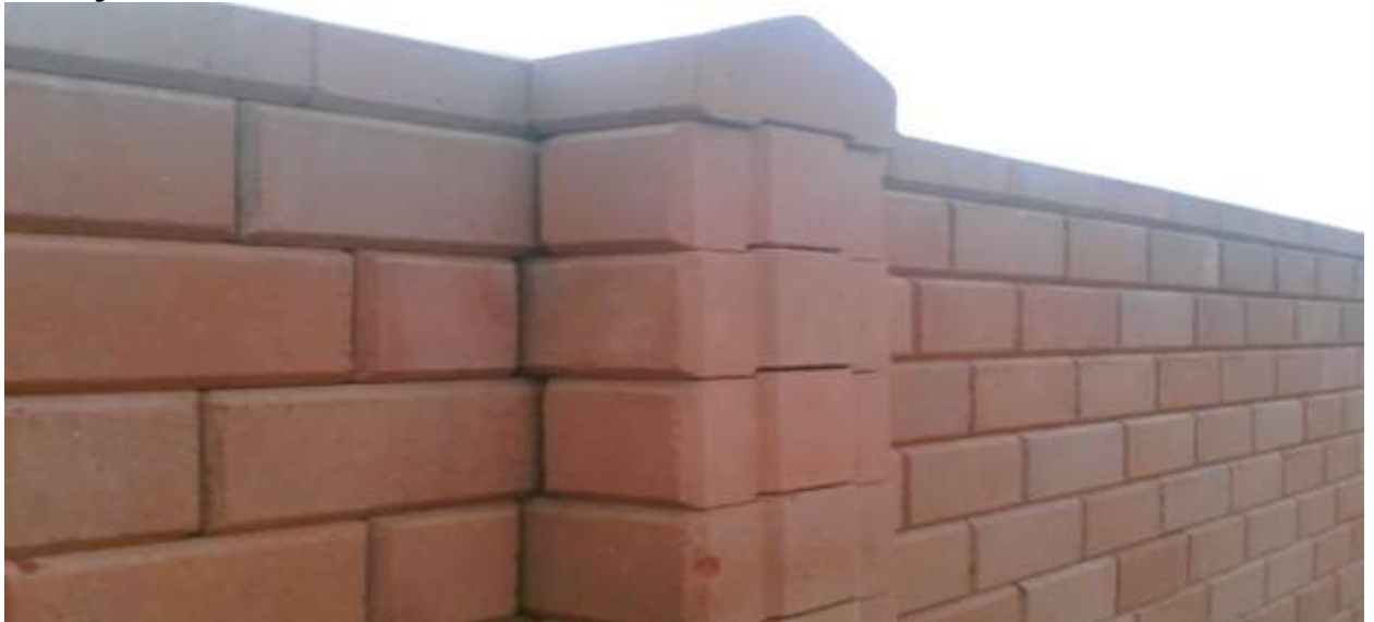
PLATE 3: A fence constructed with Interlocking Stabilized Earth Blocks
