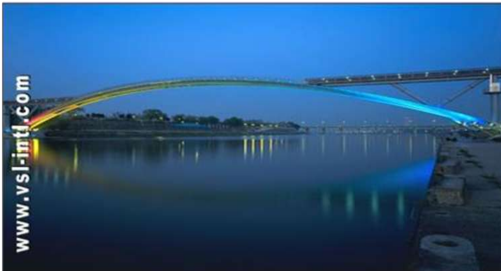
Figure 7: 120m Foot Bridge Build with UHPC in South Korea ( www.vsl-intl.com )
