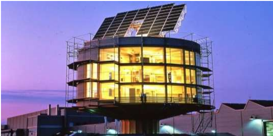
Fig 5.1.1: The spinning, sun-chasing Heliotrope designed by Rolf Disch. It can generate up to five times as much power as it needs to operate. The home sports a giant angled solar array on the roof and the entire structure is mounted on a pole timed to rotate 180 degrees each day as it follows the sun.
