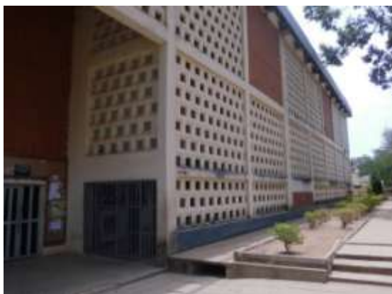
Plate ii. Shading devices Multipurpose Auditorium, University of Jos
