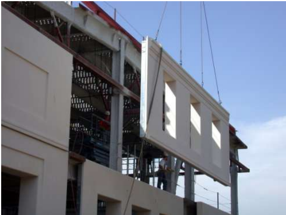
Figure3: Showing Modular Sections
