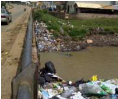
Plate 3 final disposal point for waste for local waste collectors
