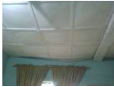
Figure 7: Sagging ceiling
