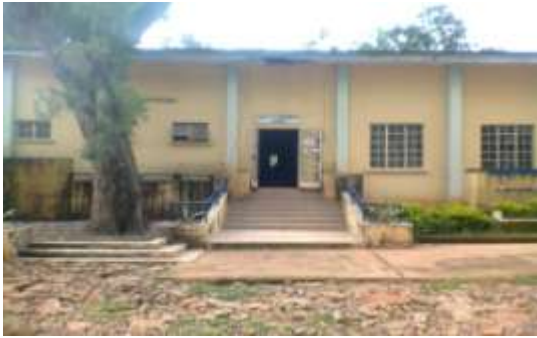
Figure 4: .Side of Building A
