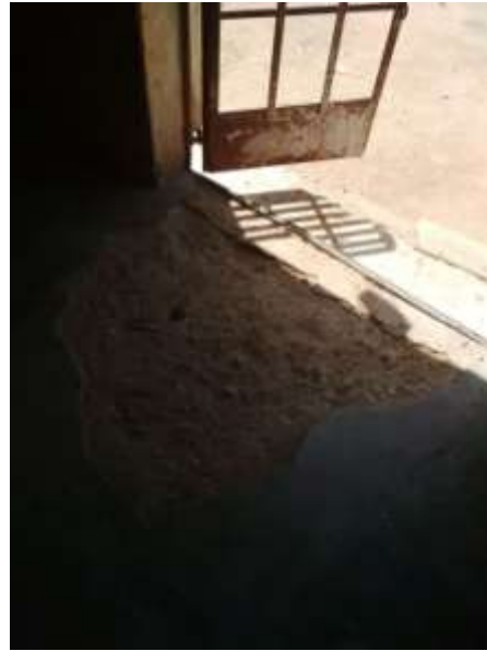
Plate v: Broken floor at threshold
