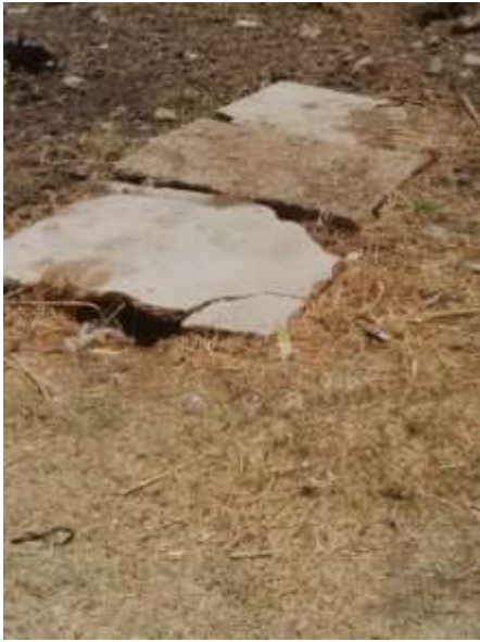
Plate iv: Broken and overflowing septic tank
