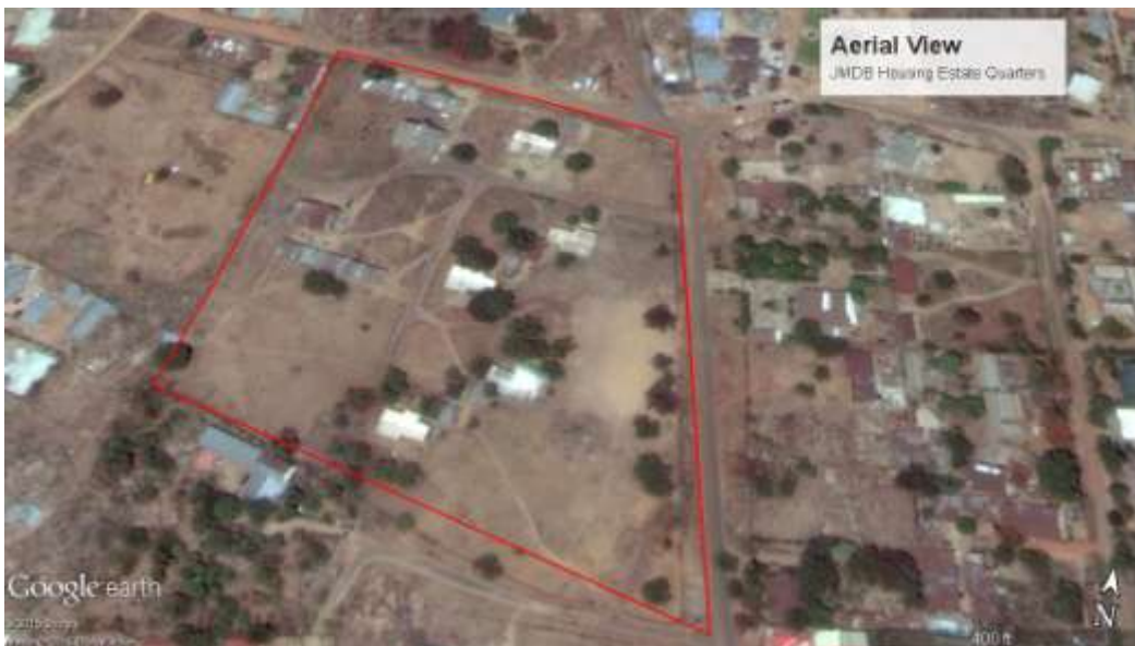
Plate i: Aerial View of study area Source: Google Earth (2018)
